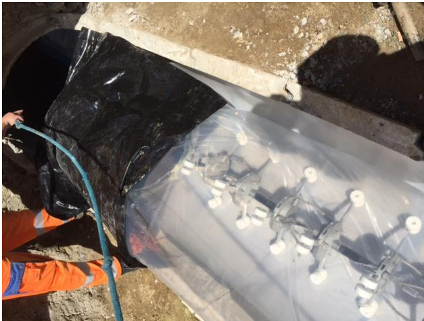
Fig. 52 Installation airlock
