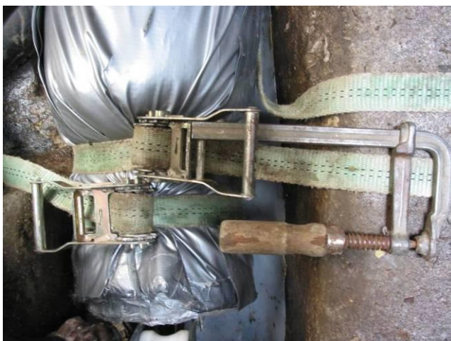
Fig. 47 Re-tightening the tie-down straps
