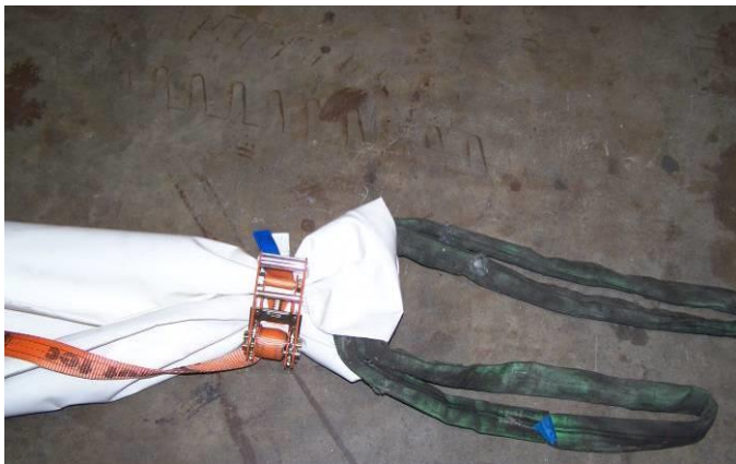
Fig. 22 Fixing the preliner with tie-down straps
