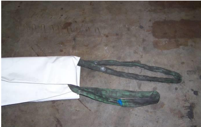
Fig. 21 Folding the preliner
