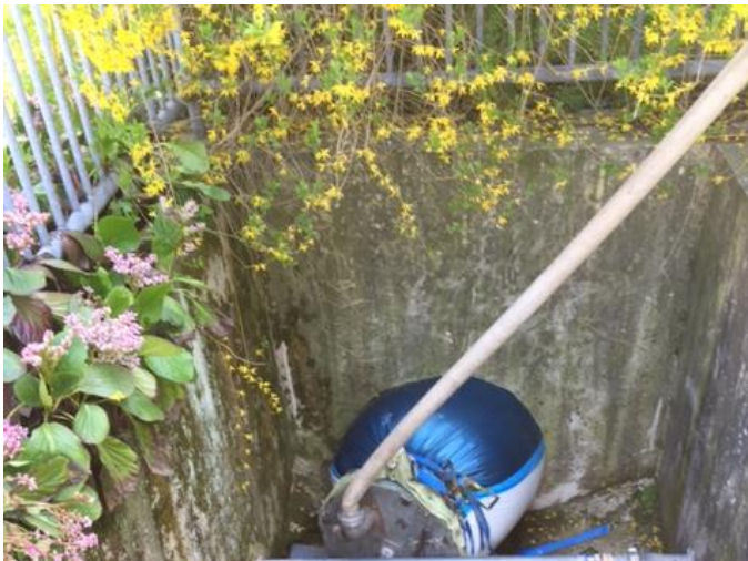
Fig. 39 Packer with tie-down straps
