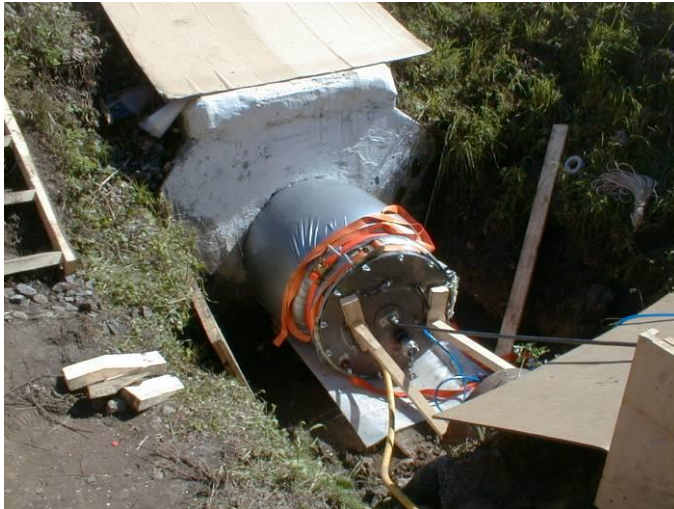
Fig. 56 Installed packer
