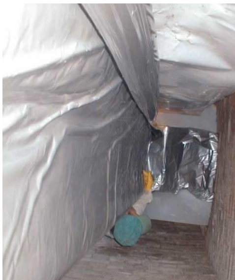
Fig. 31 Drawing the folded pipe liner into the conduit
