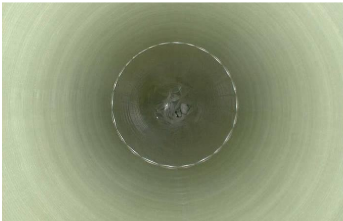
Fig. 67 Removal of the inner foil
