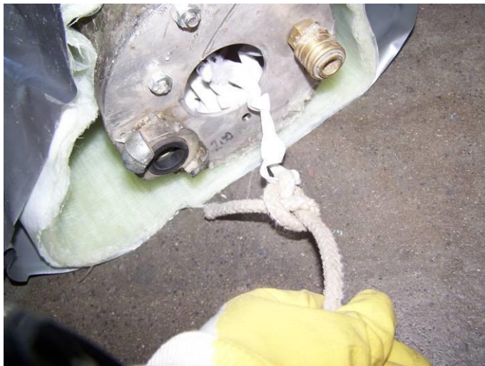
Fig. 37 Rope in packer
