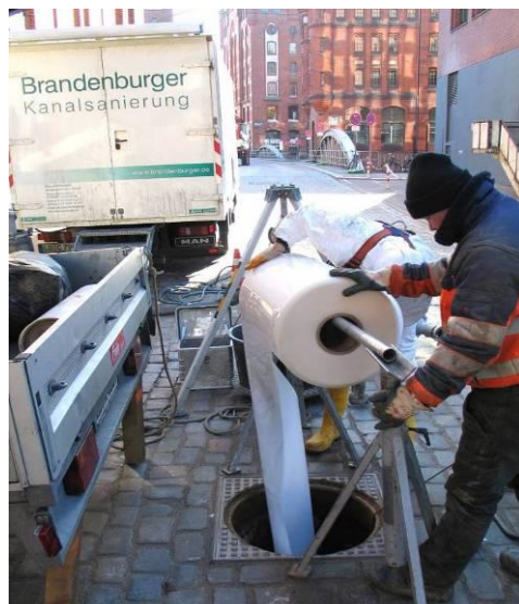
Fig. 9 Positioning the sliding protective foil at the shaft
