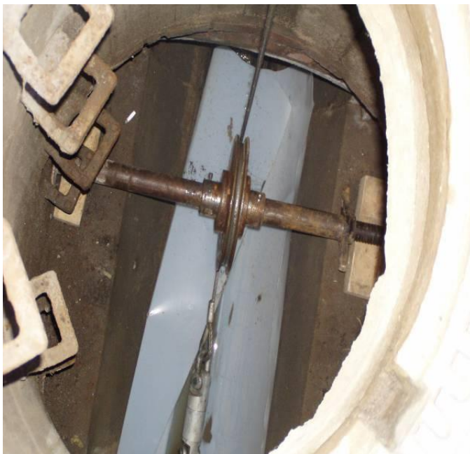
Fig. 34 Winch cable of the winch on the guide pulley
