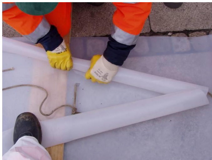
Fig. 13 Rolling up the sliding protective foil
