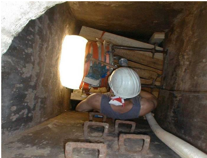
Fig. 59 Light source, at the packer
