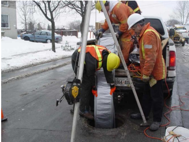
Fig. 30 Liner draw-in from the transport box
