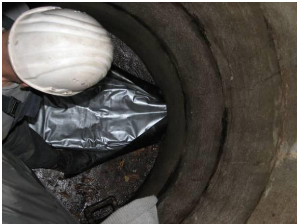
Fig. 8 Draw-in protection at the start of the pipe
