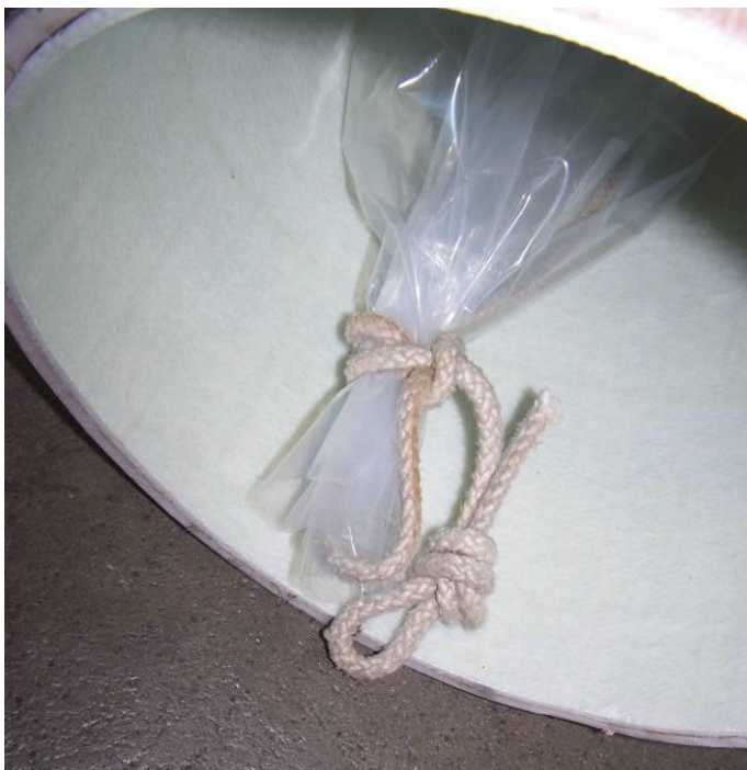
Fig. 65 Inner foil secured to the curing rope
