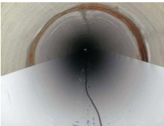
Fig. 18 Sliding protective foil in the circular profile sewer
