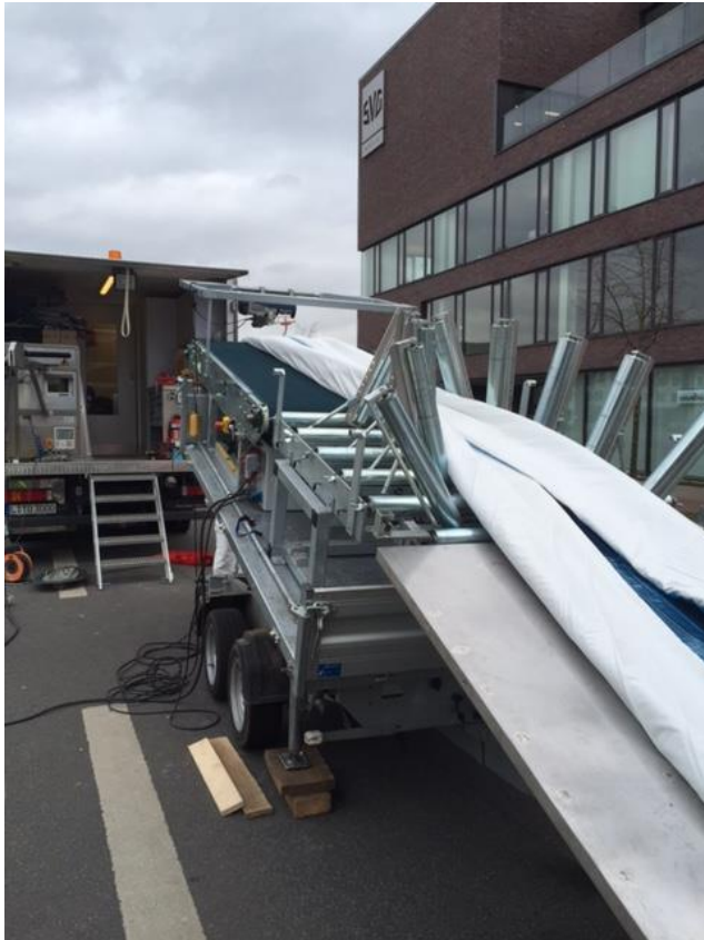
Fig. 33 Liner draw-in using conveyor belt
