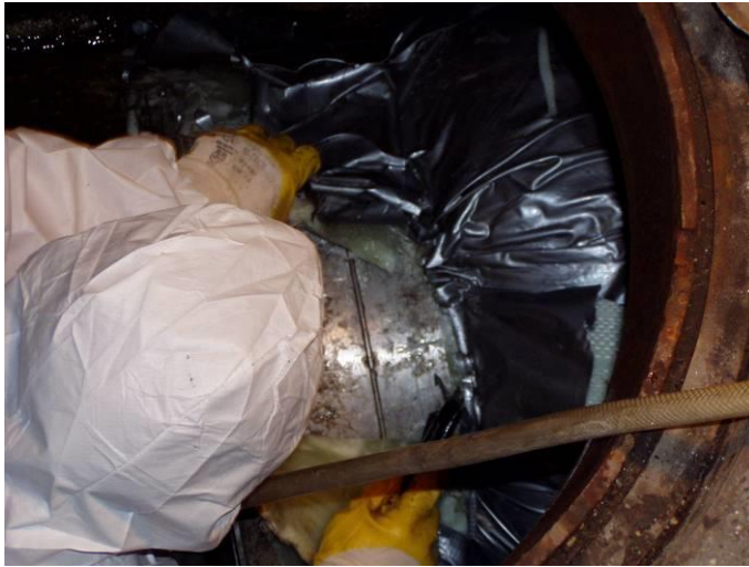
Fig. 60 Splitting the liner
