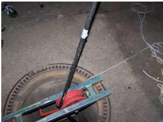
Fig. 54 Tape marking on curing cable
