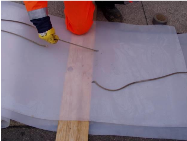
Fig. 12 Threading the curing rope
