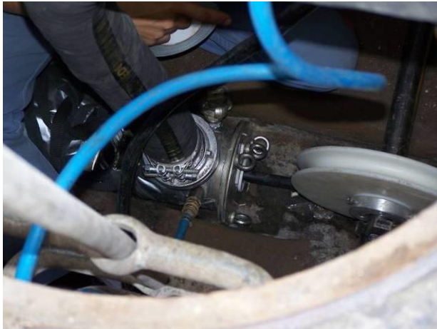
Fig. 46 Connection of packer – condenser/compressor
