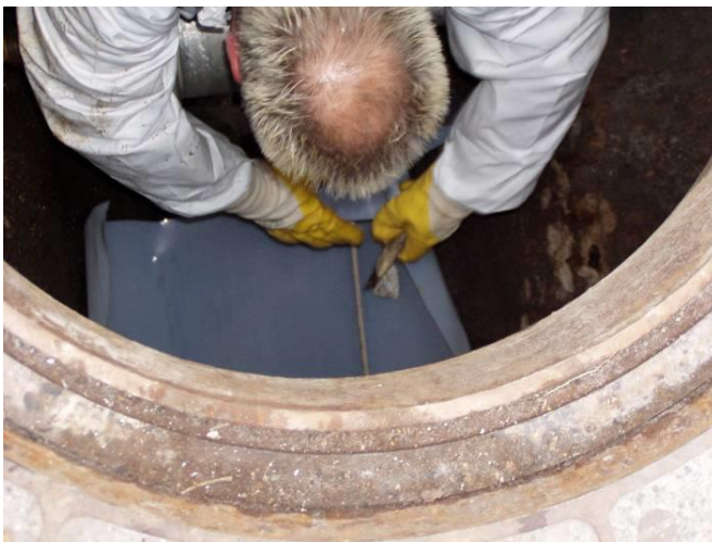
Fig. 17 Sliding protective foil in the winding shaft
