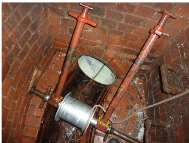
Fig. 6 Guide pulley, fastened
