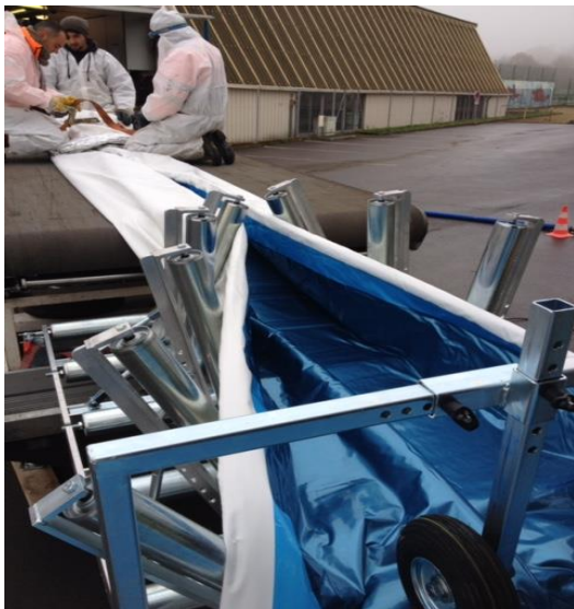
Fig. 27 Folding the liner
