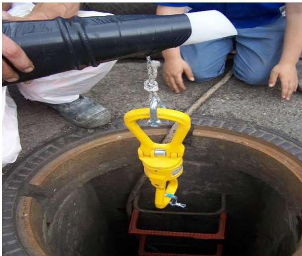
Fig. 15 Winch cable on the sliding protective foil
