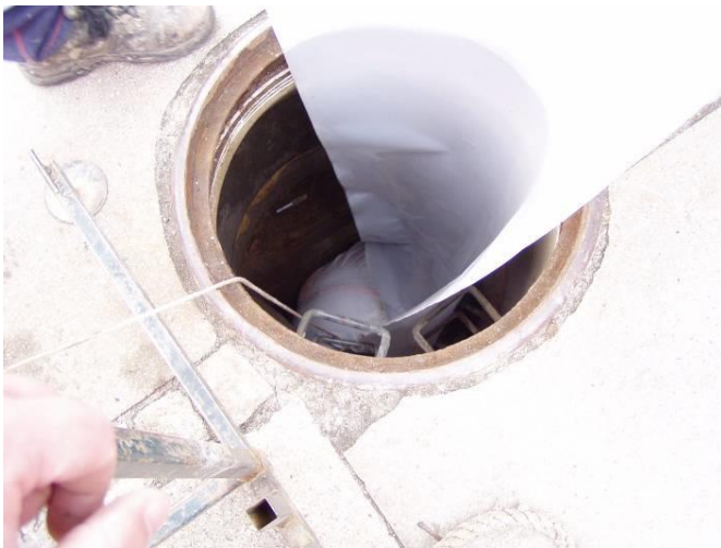
Fig. 16 Inserting sliding protective foil and curing rope
