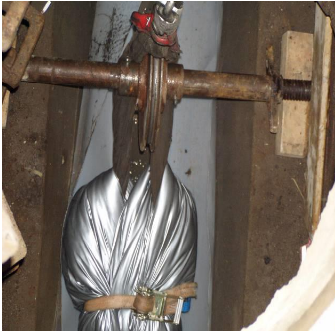
Fig. 35 Draw-in liner in the shaft
