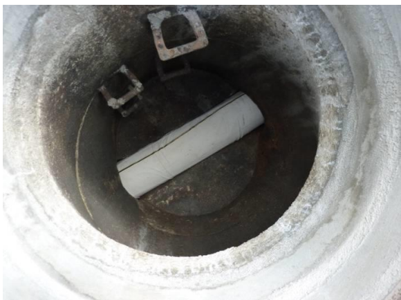
Fig. 53 Support cap with closing option in intermediate shaft
