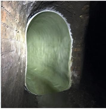
The BB<sup>2.5</sup> is available in all nominal widths. The unique design of the applied glass mats creates a high strength of the material. Even with the highest static requirements and the thinnest possible liner, a suitable variant can be selected.
