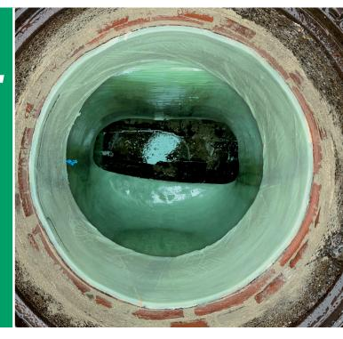
The BB<sup>2.5</sup> VERTICAL is the first manhole liner on the market, that can be securely cured with both – gas discharge technology and LED. It adapts to the prevailing manhole geometry and thus eliminates the need for time-consuming measurement.
